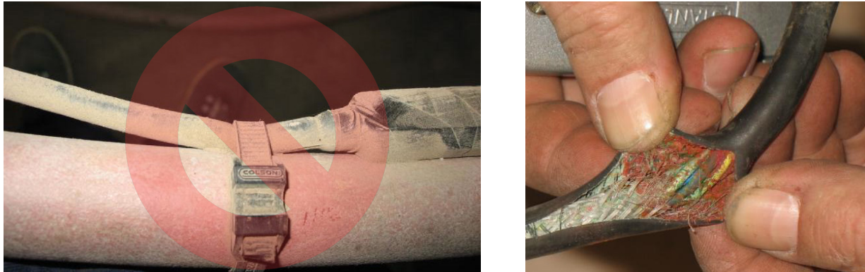
Figure 15. Do not use Zip-Ties Directly on Cables
